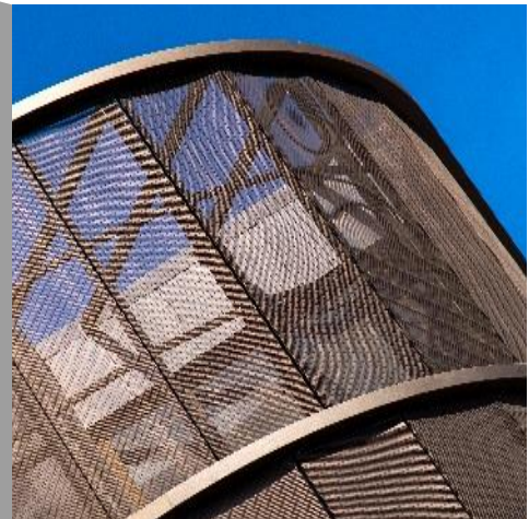
* Typical Architectural Installation
