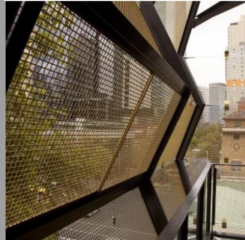
* Typical Architectural Installation
