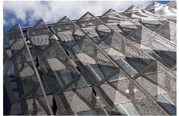
* Typical Architectural Installation of Perforated metal with varying hole sizes
