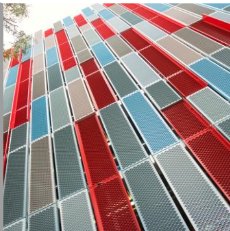
* Typical Architectural Installation
